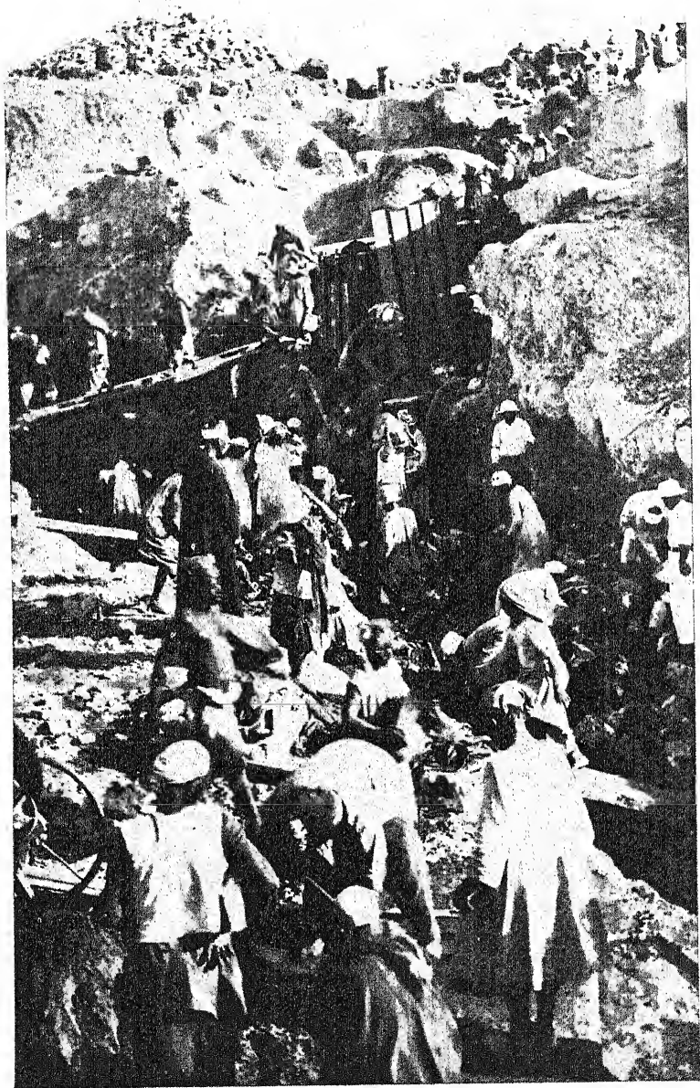
A CANAL IS DUG
